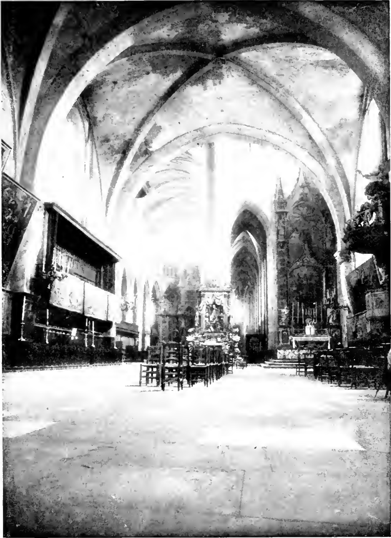
“THE NAVE OF THE XIII CENTURY IS AN AISLE-LESS CHAMBER, LOW AND BROADLY ARCHED.”—TOULOUSE.
